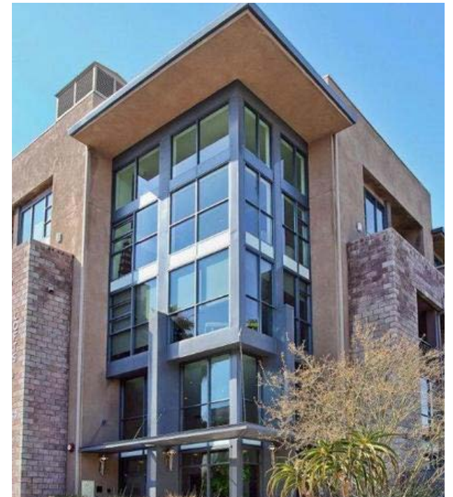
Figure 3-38: Enhanced fenestration as focal point
