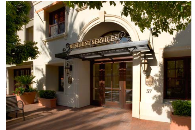
Figure 3-43: Private resident serving facility
