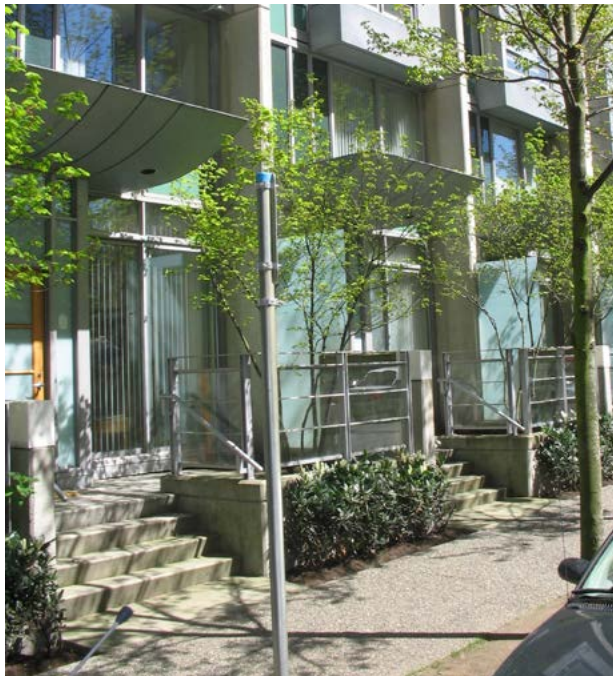
Figure 3-61: Building elevated above street level
