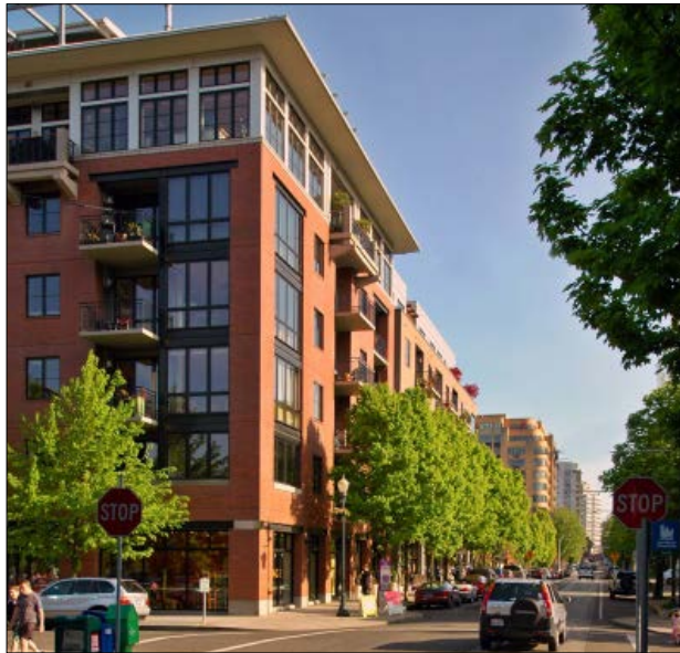
Figure 3-5: Building defining and activating the street edge
