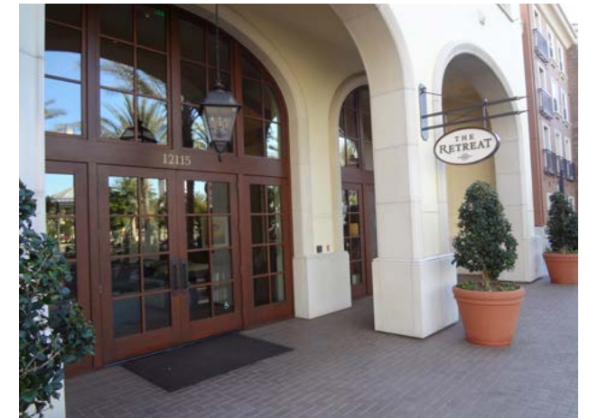
Figure 3-44: Private resident serving facility
