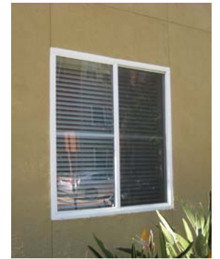
Figure 3-89: NOT ALLOWED - Flush windows without trim or adequate detailing
