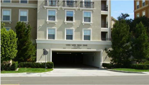
Figure 2-30: Entrance to at-grade structured parking
