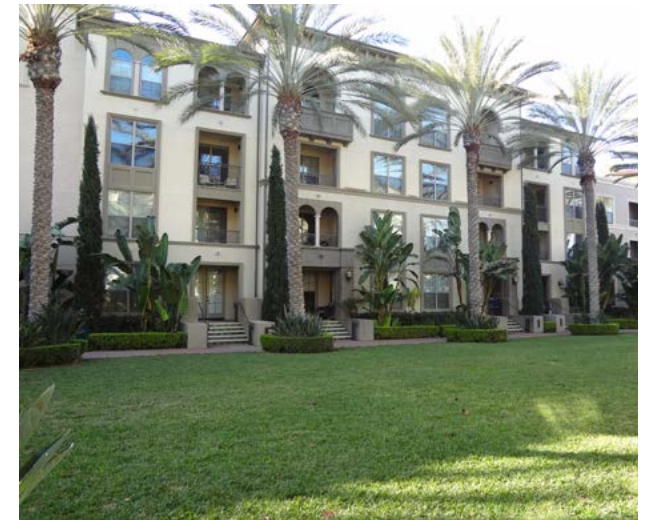
Figure 3-20: Building defining park edge
